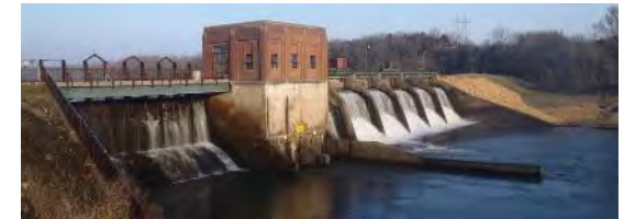
Maquoketa hydroelectric power plant. Photo Credit: http://renewableworldenergies.com
